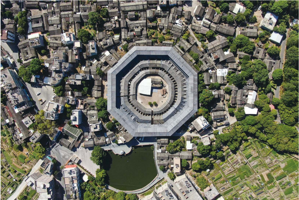
Photo taken on October 21, 2022 shows Daoyun Lou, an octagonal Tulou earthen building compound in Raoping County of Chaozhou, south China's Guangdong Province. Daoyun Lou, which covers a floor area of 10,000 square meters, is China's largest octagonal Tulou earthen building discovered so far. In 2006, it became a major historical and cultural site protected at the national level. ( Xinhua/Deng Hua )
